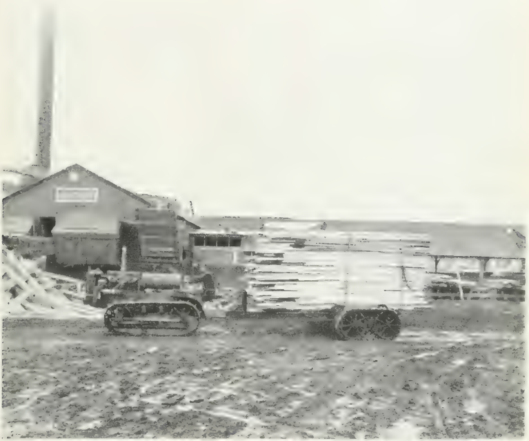
FIG. 146. CATERPILLAR IN LUMBER YARD.
